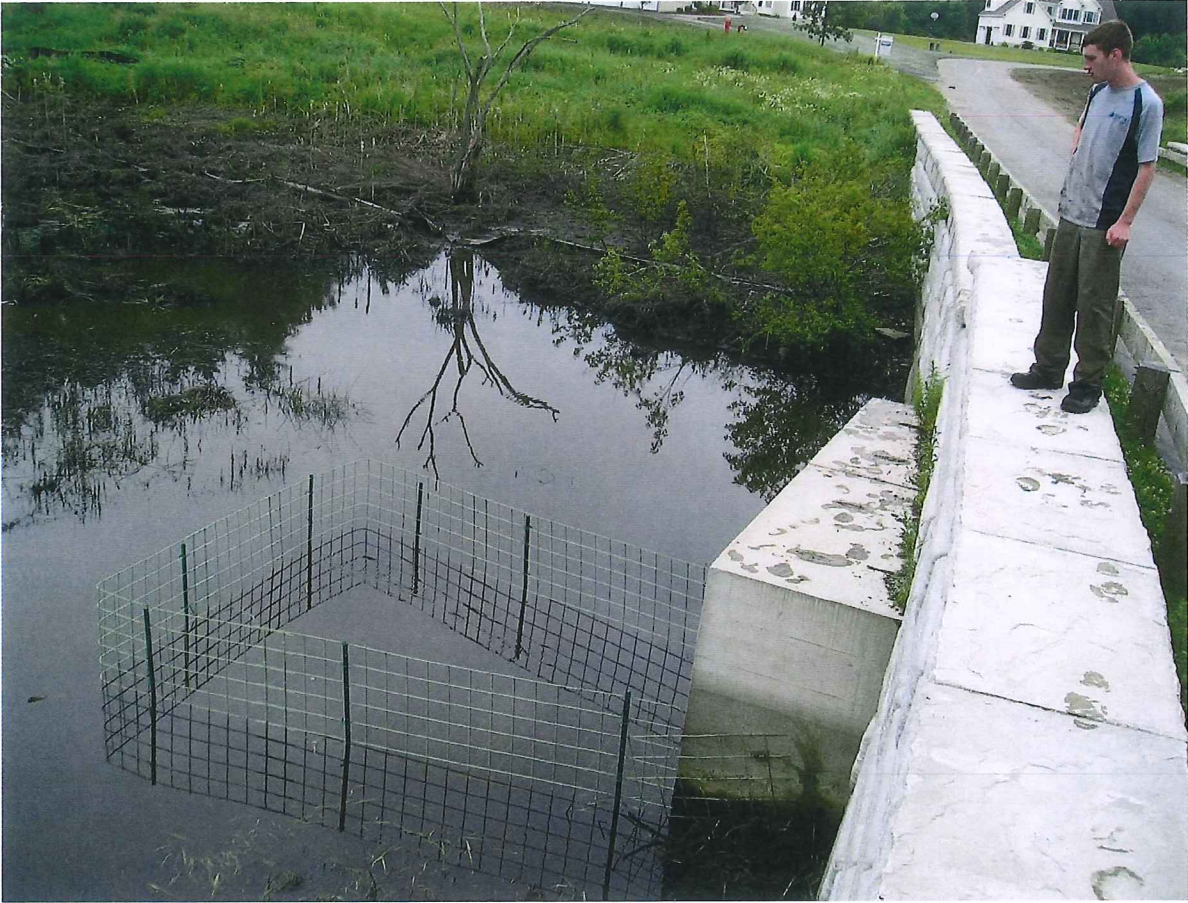
Trapezoidal protective fence installed after re-opening dammed culvert
