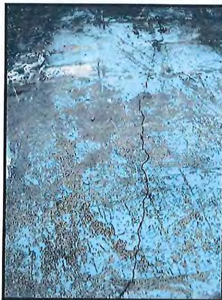
Photo 1 – Typical Hairline Cracking in Concrete Slab
