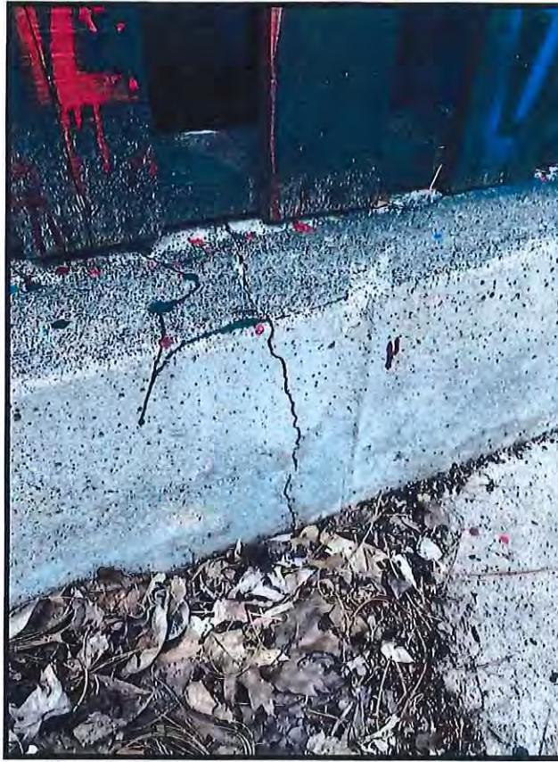
Photo 3: Enlarged view of Foundation Wall Crack
