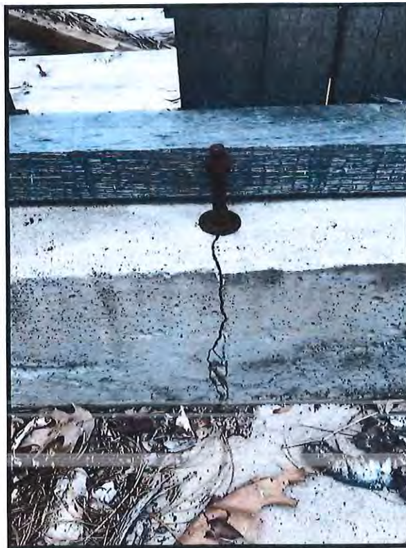
Photo 2: Bent Anchor Bolt & Foundation Cracking
