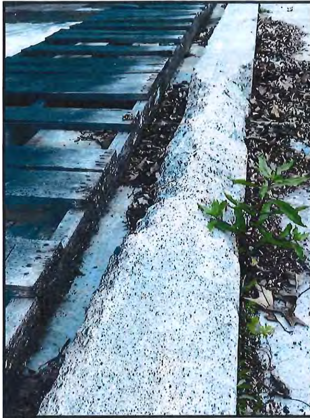
Photo 4: Portion of Foundation wall to be Replaced
