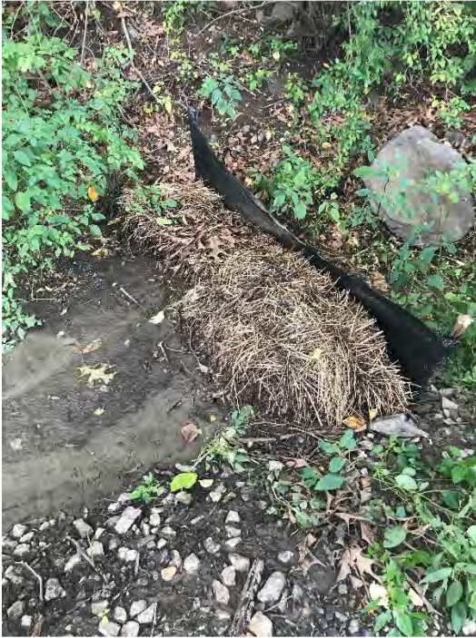
Photo 1: Silt fence/haybale barrier @Lathrop Lane
