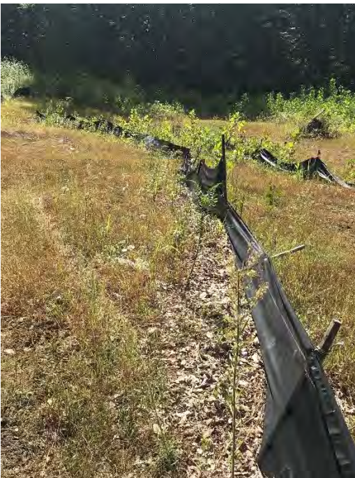
Photo 3: Hole #15 upgradient E&S controls
