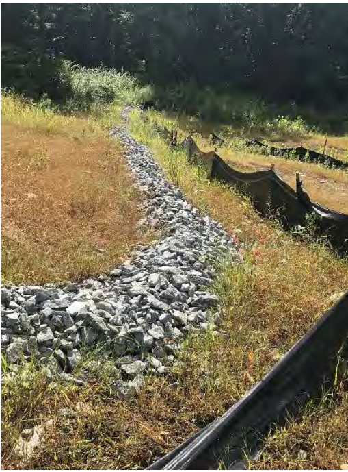
Photo 4: Hole #15 down gradient E&S controls
