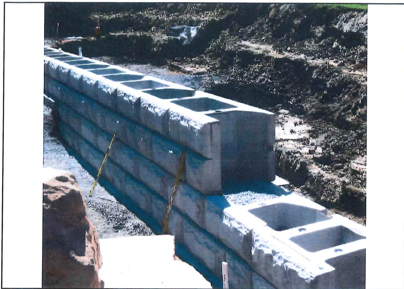
Photo 1: Typical backfill trap wall installation
