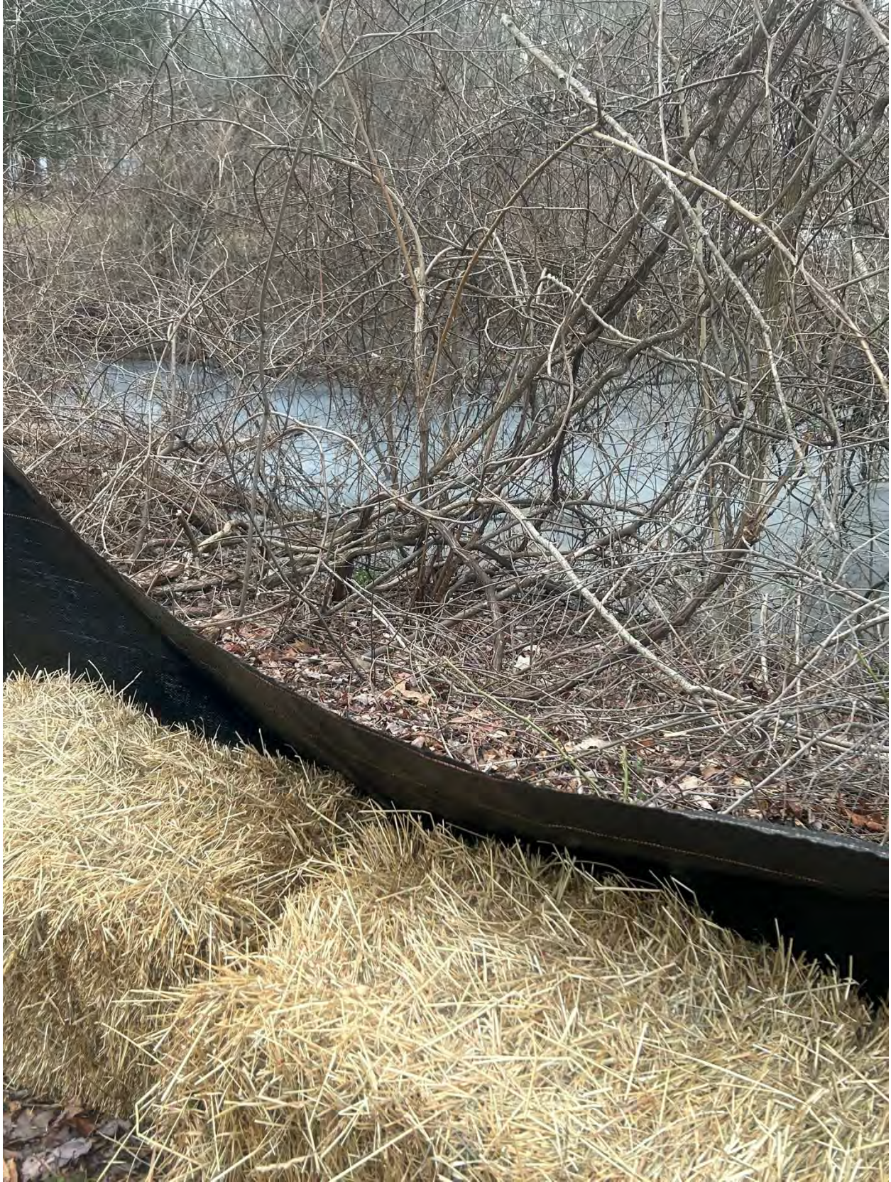
Photos shown Silt fence and hay bales
