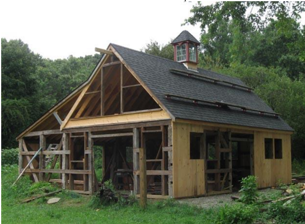
Roof in place, cupola added and barn is ready for siding
