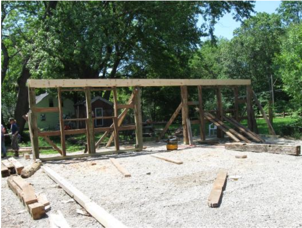
Bent erected and sills in place
