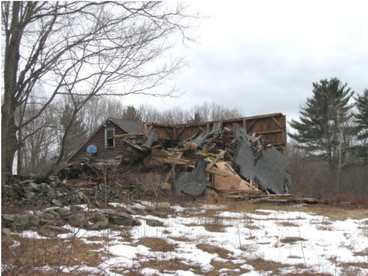
Barn collapsed under the weight of heavy snow 2011
